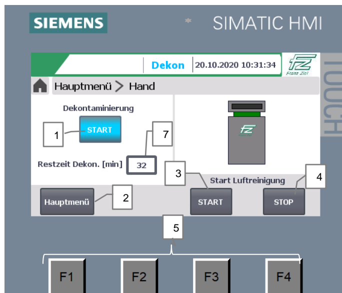
Fig. 5-7: Start of decontamination
